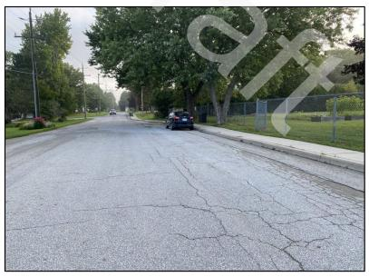
Alice Street is a local road consisting of a 2-lane cross section with an assumed (unposted) speed limit of 50 km/h. One "SCHOOL AREA" (Wc-1) Sign is installed about 70 m north of Campbell Street, although no crosswalk exists at this location. There is an
