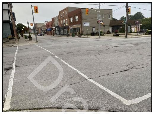
Local industrial activity in Markdale results in significant turning movements by trucks at the Toronto Street / Main Street intersection. To facilitate these movements the stop blocks are set well back from the intersection. The location of the stop blocks may result in increased speed for turning vehicles, as well as compromised sight distances for such movements.
